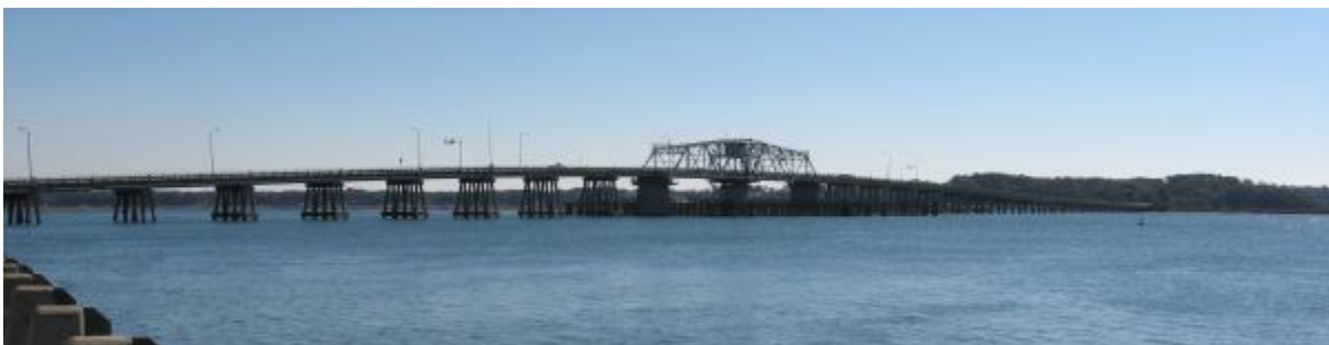
Contemporary bridge span from Beaufort to Lady's Island
